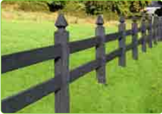
150mm x 150mm posts, 150mm x 44 rails
