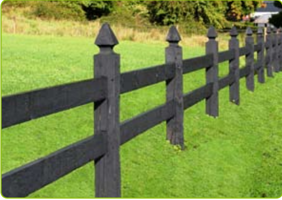
150mm x 150mm posts, 150mm x 44 rails
